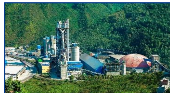
Xunyang Plant, Southern Shaanxi
