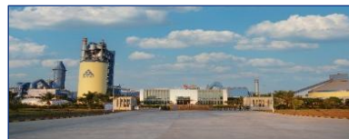
Dugongo Cement, Mozambique
