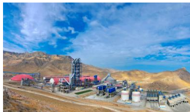
Uzbekistan - total capacity: 2.5mt
