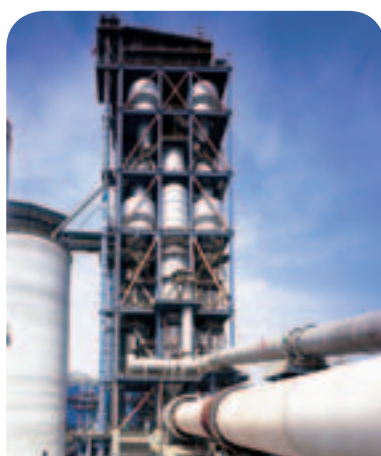
Ankang is West China Cement's third cement plant to come online, following Pucheng and Lantian
