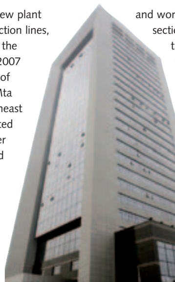
West China Cement Ltd's headquarters building in Xi'an, provincial capital of Shaanxi Province
