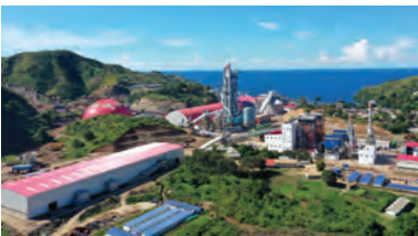
Great Lakes Cement Plant, DRC
