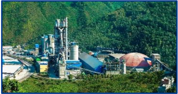
Xunyang Plant, Southern Shaanxi
