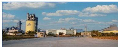
Dugongo Cement, Mozambique
